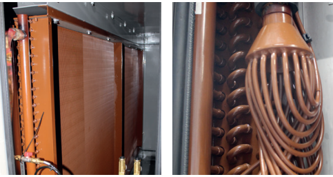
Herasite protection on the entire battery and support frame
